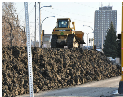
Building of 2 nd St. Levee for 2009 Fargo-Moorhead Flood
